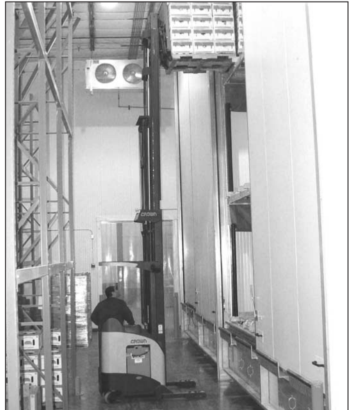
The flexible design of the PalletFridge™ allows easy loading and unloading in an aisle only nine feet wide. Boulder Fruit Express - Denver, Colorado.
