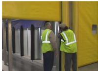
In rooms equipped with fabric doors, inspect roller mechanism to make sure door is sealing smoothly and evenly along each side. Repair or replace Velcro as needed if excessive bunching or gaps appear. Tears can be repaired using same color vinyl tape on the inner and outer sides of the tear.
