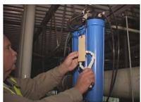
Access and visually inspect all filters in the reverse osmosis system. Replace filters as needed based on local water quality, but at least once per year. Follow all instructions for system care and maintenance. Place a tag on the system to keep track of service dates and filters exchanged.
