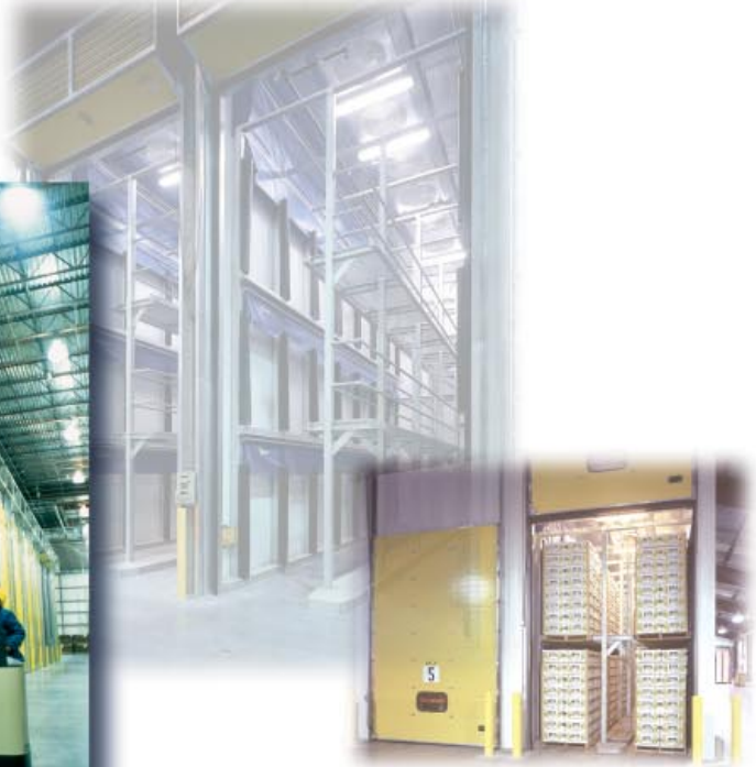
Two-tier, dual entrance, 44 pallet TarpLess® Ripening Rooms. Safeway Distribution Center, Portland, Oregon.
